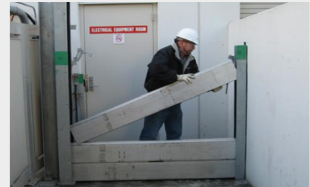
Deployable stop logs to protect vulnerable entryways
